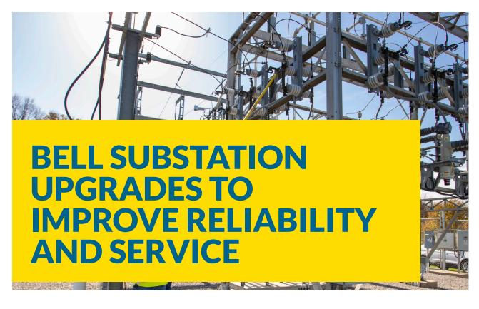
Substations play a critical role in the electric grid by facilitating the transmission and distribution of electricity from power plants to homes and businesses. They are responsible for changing the electrical voltage from high transmission levels to lower distribution levels, enabling the safe and efficient delivery of electricity to end-users. Substations also provide a way to manage the flow of electricity, ensuring that power is delivered where and when it is needed.
