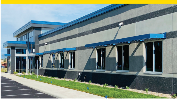
Sturdy, pre-cast concrete panel exterior.
