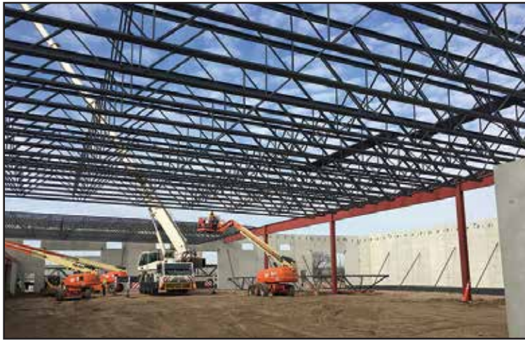
The steel trusses were installed in the garage and warehouse portions of the facility in November.
