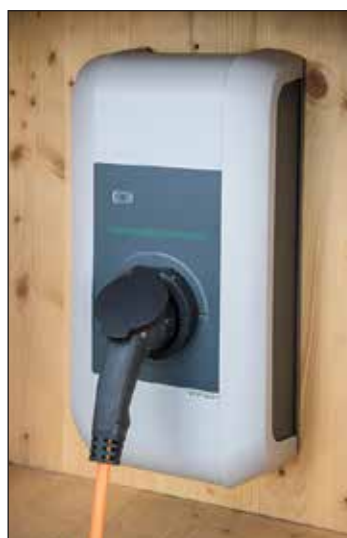
This is a 240-volt outlet for a Level 2 charging unit.
