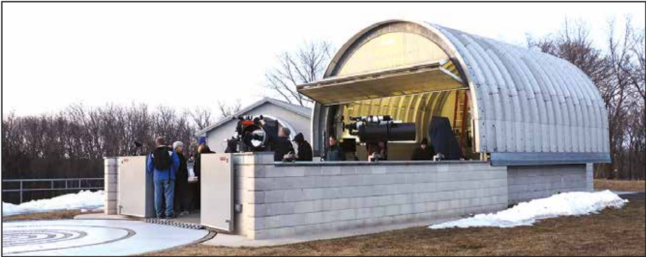
The Onan Observatory has a roll-off roof with a “three short-barreled shells” design, which retracts for outdoor viewing on fair-weather nights.
