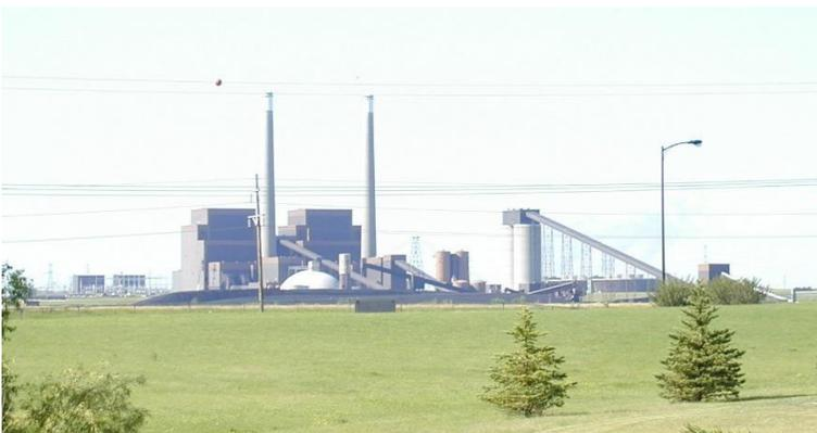
Coal Creek Station, near Underwood, ND provides baseload power using clean-coal and Dry-Fining™ technologies. The two units of Coal Creek Station have over 1,100 MW of generating capability. The extensive walking tour through the power plant is very educational and views from the 21<sup>st</sup> floor observation area are phenomenal.
