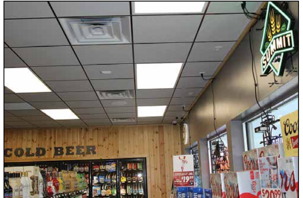
LED fixtures replaced incandescent lighting in the ceiling and refrigerator. Even the beer lights have been replaced with LEDs.
