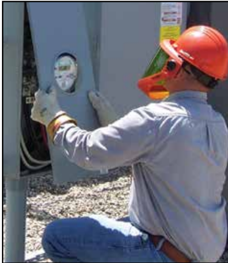
energized meter must be done by a trained Co-op employee using the proper protective equipment.
