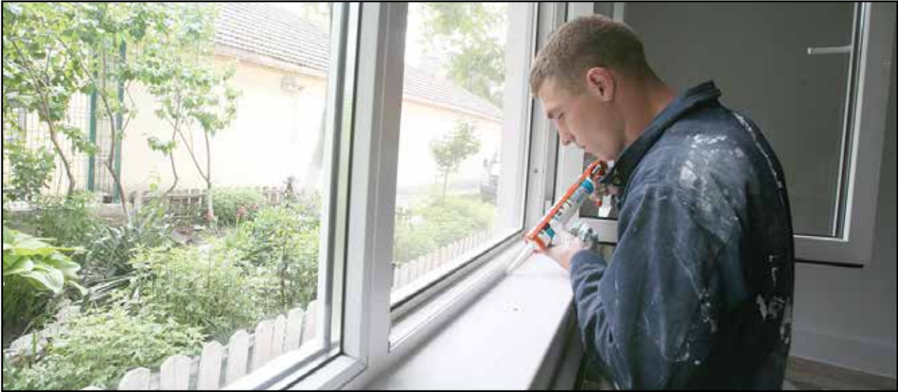
Sealing air leaks is critical to keeping the home’s interior cooler than the exterior. Source: Wikipedia Commons (no attribution required)
