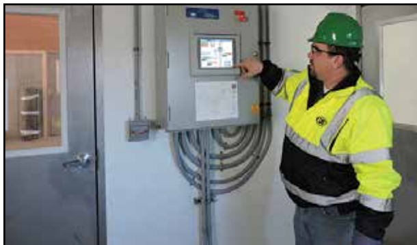
The plant is completely automated. Crop Nutrition Operations Manager Aaron Schwab can automatically select a bin for a train car's contents to download into. The touch screen allows the office to view the same information as the receiving area.
