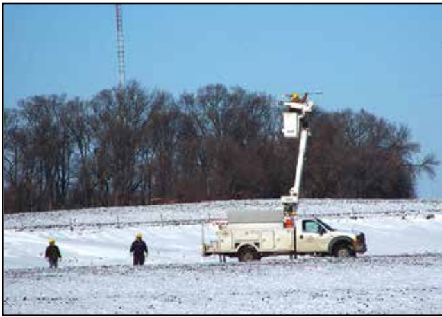
Lineman from Hutchinson Utilities assisted McLeod Co-op with system repairs. They are restoring lines across a farm field north of Hector.
