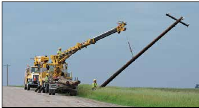
MCPA line personnel carefully guide large 3-phase pole into new hole that was dug after snapped off pole was removed.
