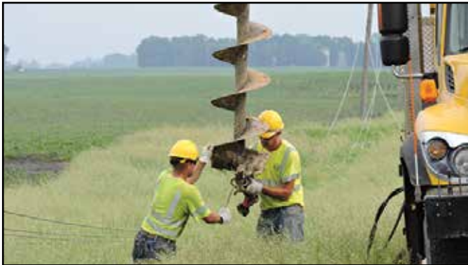
MCPA linemen make repairs to auger before work of digging a new hole can begin. Linemen have to use mechanical skills daily for assembling hardware and mounting it on crossarms, mounting crossarms onto poles, and making equipment repairs of all kinds.
