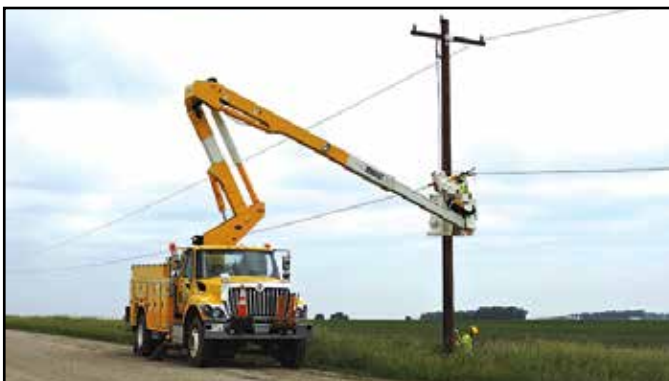
A MCPA line worker in the bucket puts the second conductor of a 3-phase line back up near Buffalo Lake.
