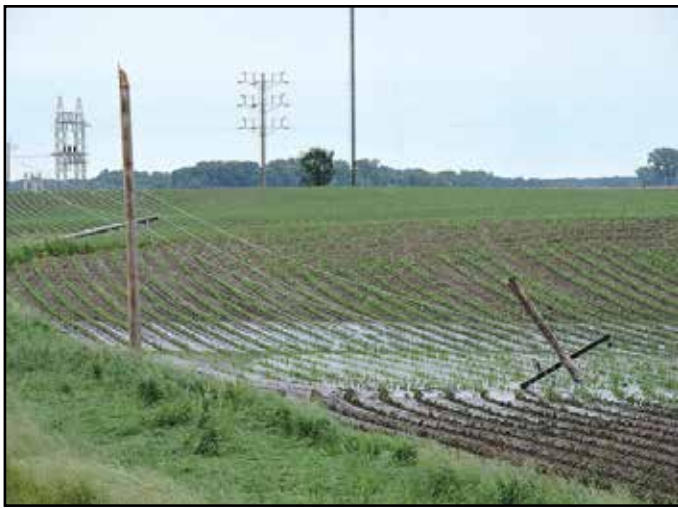
Straight-line winds on June 11 snapped off many power poles along one stretch of roadway, leaving the tops of poles in a farm field and conductors blocking one member's driveway.
