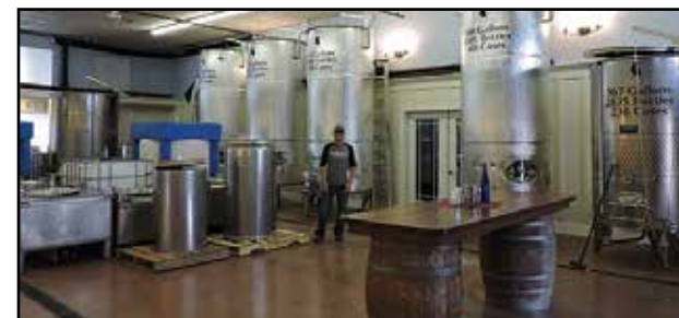
The fermentation tanks are used to produce the various wines. The wine is also cooled in the tanks to 28 degrees (but it does not actually freeze). The cooling system is similar to a bulk tank cooling system used in a dairy operation.
