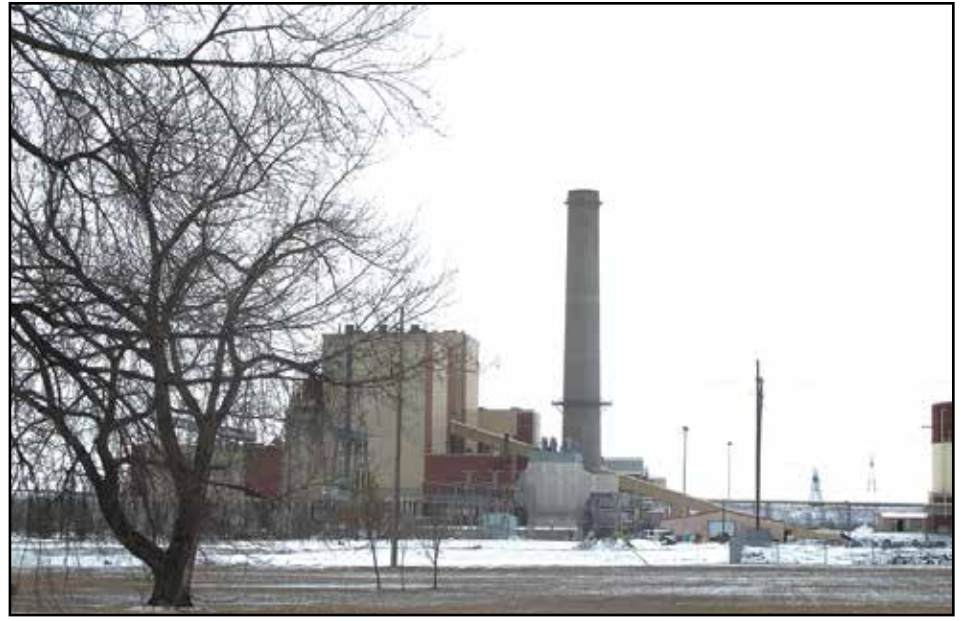
Great River Energy's Stanton Station, after celebrating its 50th anniversary a few months ago, went out of service on Saturday, February 25, marking the end of an era for a plant that has been part of the Stanton, ND community for generations.
