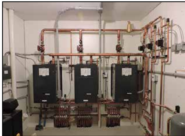
The mechanical room contains three 54 kW three-phase boilers. The boilers are manufactured by Electro Industries. The boilers operate as one unit, even though they supply multiple heating zones that have different thermostat settings.
