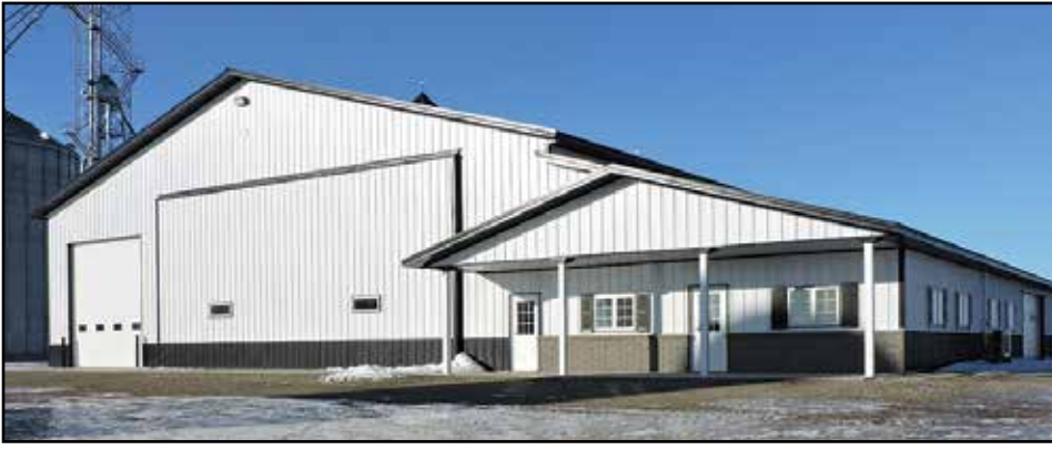
The 12,000 square foot farm shop and office is heated on the Co-op's off-peak electric rate. It utilizes three electric boilers that heat and circulate water at night from 11 p.m. to 7 a.m. on the Storage Heating Program. The 12" of sand beneath the cement slab stores enough heat to keep all areas of the shop and office warm 24 hours a day.
