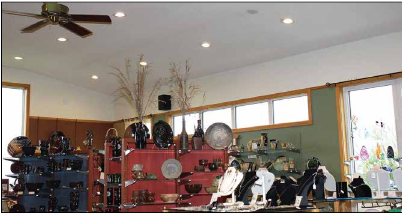
Switching to 35 LED can lights from 121 halogens cut energy use by 95% in the Gallery. The Gallery contains hand-made art from 150 artists from across the country. It's a one-stop Gallery for special occasion gifts.
