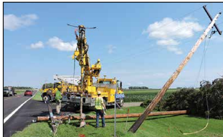
MCPA crews replaced a power pole broken off during the August 4 storm.
