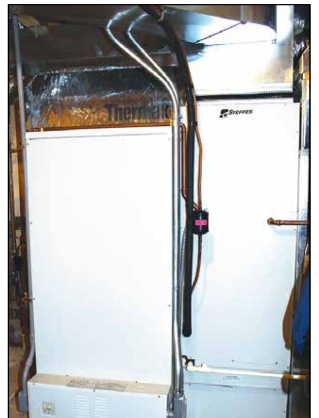
A Steffes storage furnace heats bricks at night and radiates heat all day.
