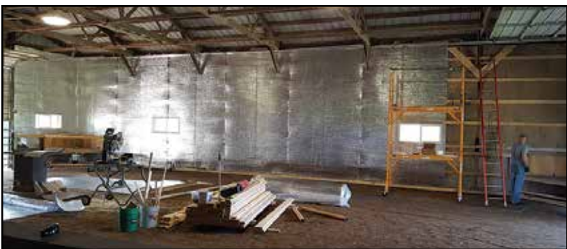
Insulation work that has been completed over the summer in the riding arena. Lighting, ventilation, sheet metal work are yet to be finished.
