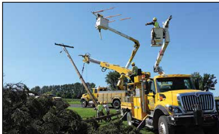
Trees falling over or into power lines caused many of the outages on August 4. It takes additional time for crews to make repairs to electrical equipment when they have to cut and clear trees away first.
