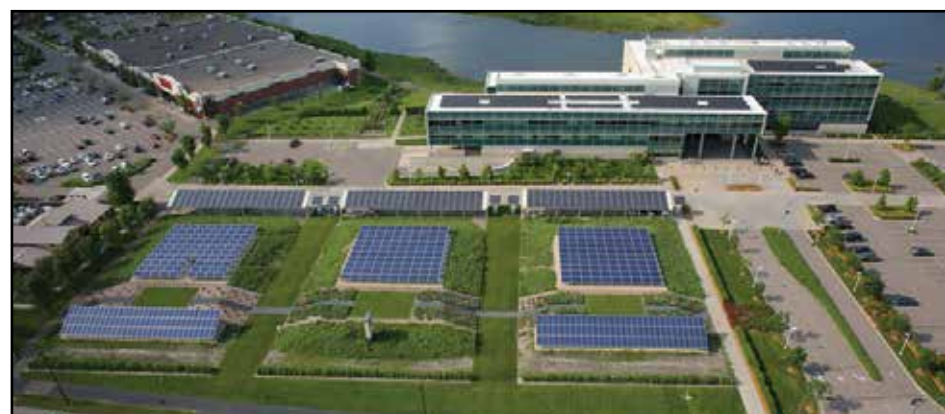
250 kW array at GRE's Maple Grove headquarters
