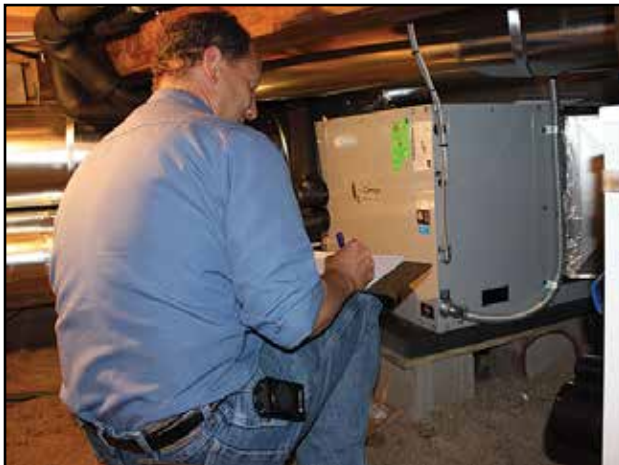
A GSHP can be installed even in a crawl space, like this unit installed under a lake cabin.
