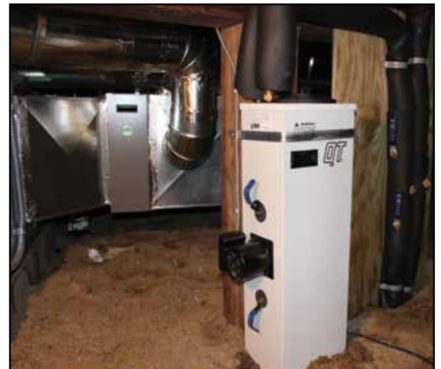
This is a forced-air unit. However, GSHPs can also be used to provide radiant water heat, either baseboard or underfloor.
