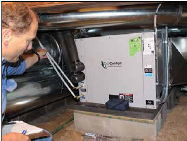
Energy Management Technician Allen Lendt does a "check out" of the system to make sure it is set to deliver low-cost heat and air.
