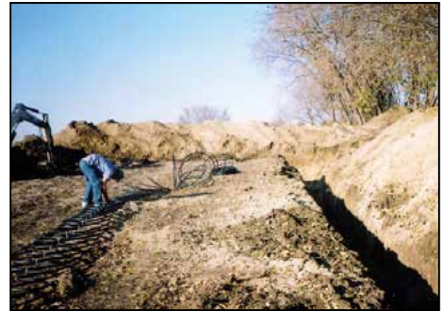
The old way of installing tubing involved digging trenches and laying the tubing into the trench, which was invasive and more expensive.
