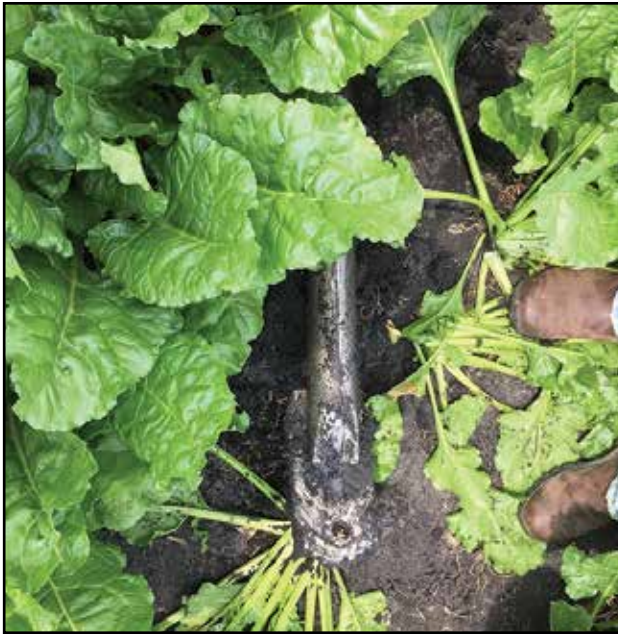
The hole on the end of the pipe will accept the geo thermal tube (right). As the pipe is retracted, the tubing is pulled through the bored holes.
