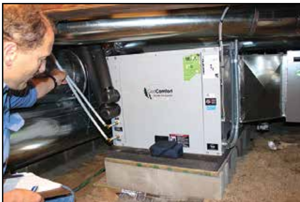
Meeker Co-op Energy Management Technician Allen Lendt checks out a geo thermal unit installed in a crawl space under the Stubson's Lake Minnie Belle home.
