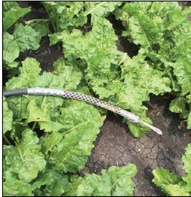
This geo thermal tube will be pulled through the bored holes in the ground. The tubes will circulate an anti-freeze mixture, drawing heat from the ground and transferring it into the home.
