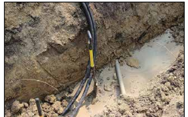
The gray pipe is boring holes through the yard and into a nearby field. The holes will ultimately be filled with geo thermal tubing.
