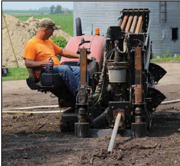
Dale Brenhaug of Mid MN Geothermal Services, Inc. using this boring machine to insert pipes through the ground, eliminating the need to disturb yards with extensive digging.
