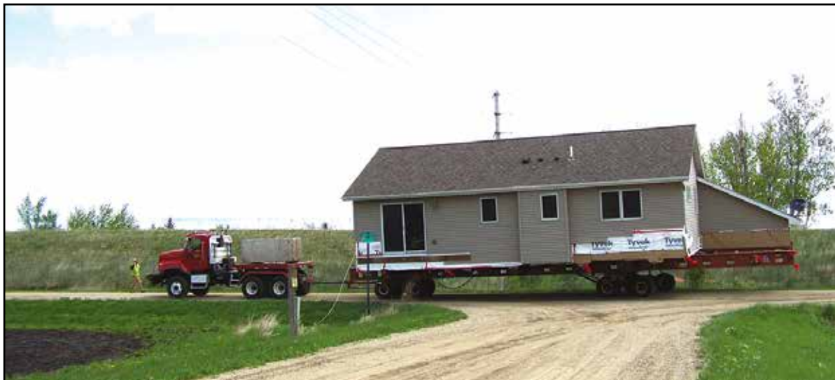
The house has clearance to move beneath the three-phase City of Glencoe power line along Lace Avenue (near Spruce Ridge landfill) because MCPA line crews had already dropped the distribution wires underneath. Wires were reconnected as soon as the house passed by.
