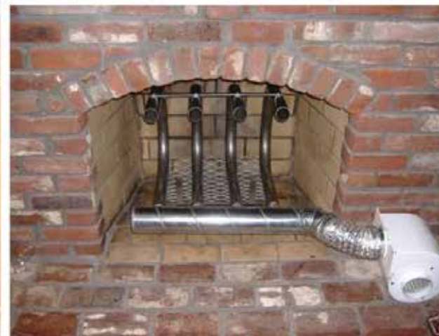
These images show various types of heat-circulating fireplace grates heating indoor air. Some grates use fans, and others rely on natural convection circulation.
