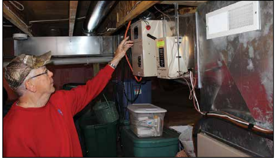
Their crawl space didn't allow the plenum heater to be installed vertically atop the furnace, so they mounted it horizontally in the duct, which works just fine.
