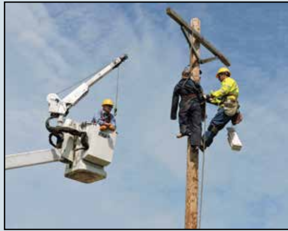
Line foreman Grant Miller watches as apprentice line worker Jared Klein tries the rescue procedure.
