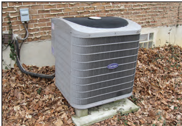
Provide adequate clearance around outdoor unit for good air flow through the coils. Photo credit - James Dulley
