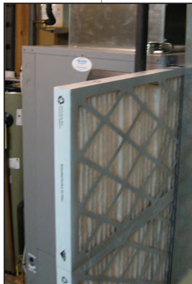
Change the air filter regularly. This is a high-quality pleated media filter. Photo credit - James Dulley
