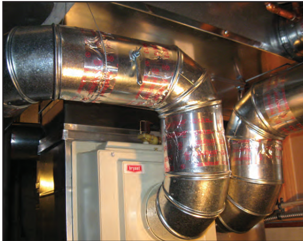
Seal duct joints with duct tape and close off the humidifier duct damper. Photo credit - James Dulley
