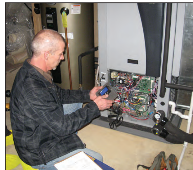
The air-conditioning system is complicated, so you need a technician to do regular maintenance. Photo credit - James Dulley
