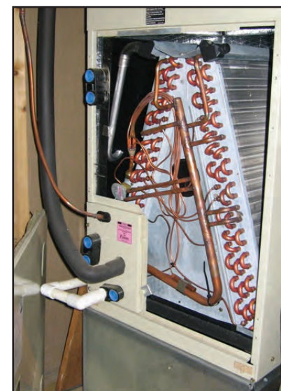
Turn off the power to the indoor unit and vacuum the blower and evaporator coils. Photo credit - James Dulley
