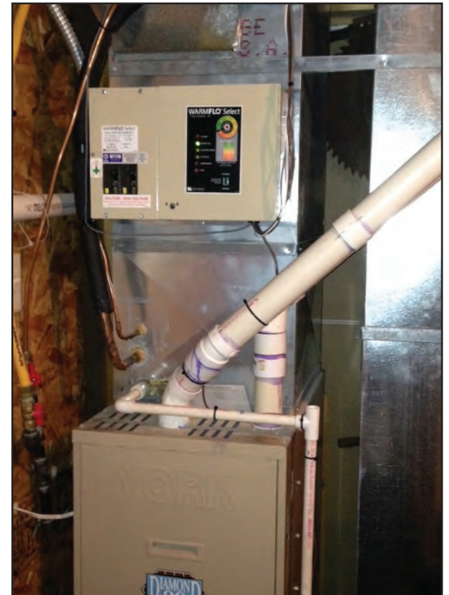
Simply adding a plenum heater to a propane furnace qualifies members for the low energy management electric rate.
