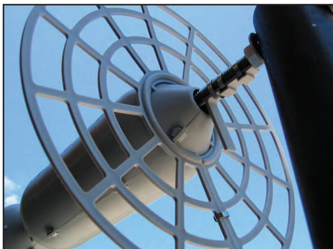
Animal guards come in all shapes and sizes. Pole-style guards in our area often look like this. While not foolproof, these guards go a long way toward protecting squirrels and reducing outages.
