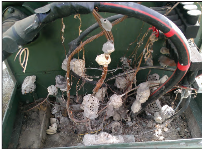
Critters of all kinds can cause a power outage, even a colony of wasps that invade a transformer.
