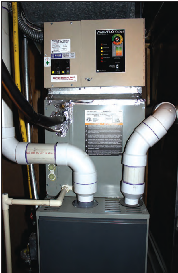
This compact unit combined with the air source heat pump unit that sits outside, heats the Lickfelt's 2,600 square foot home for $150.00 a month on average last winter.
