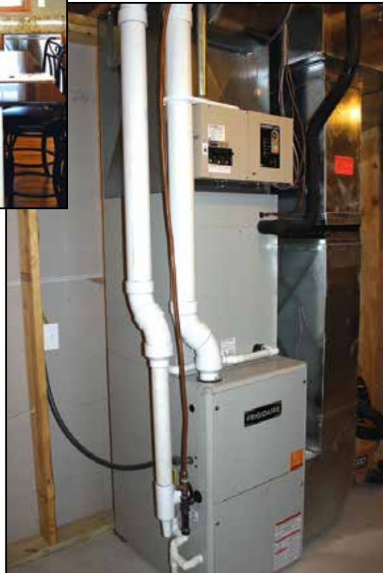
The heating unit includes a plenum heater (top), the A-coils of the air source heat pump (mid-section) and the furnace (bottom section). The heat pump unit sits outside like a central air unit. Together, this system is highly energy efficient and qualifies for the low energy management rate when controlled.
