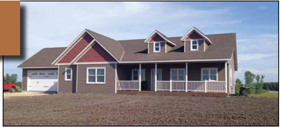
The Schwarzrock's new home in rural Hutchinson was planned to provide low-cost heating on the Storage Space Heating Program using a Steffes Central Storage Furnace that provides both hydronic (in-floor heating) and forced air heating. In the garage they are planning to use Stiebel Eltron heating mats, also on the off-peak storage heating rate. Water will be heated by a Marathon water heater on the Storage Water Heating Program. Summer cooling and fall/spring heating will be done by an air source heat pump on the off-peak rate.
