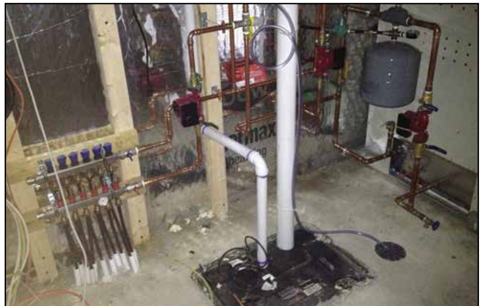
The piping going into the floor on the left includes one supply and one return manifold for six piping loops each. The piping goes down into the floor and is embedded in the concrete throughout the entire basement to provide heat as needed. (The white pvc piping has nothing to do with the heating system – it is a sealed sump pump and vent). Just above the piping is a small red and black circulating pump. That pump comes on when any of the zones in the basement floor call for heat and it sends hot water from the primary heat loop out to the floor tubing. A galvanized mixing valve is used to temper the water temperature. On the right is the primary loop. It includes a pressure tank and circulating pump. Unheated water flows into the furnace, through the hot ceramic brick, and back out as hot water that will be sent to the tubing in the floor or to the water coil in the furnace's air handler if the upstairs thermostat calls for forced air heat.
