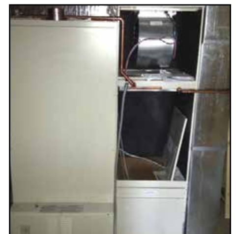
The Steffes central storage furnace is manufactured in North Dakota. It is filled with ceramic bricks that are heated electrically for eight hours in the middle of the night. The furnace is able to heat the home 24 hours a day. It can provide heat to both the in-floor basement heating and the forced air heat for upstairs. The air handler on the right will eventually include an A-coil for the air conditioning and a water coil unit to transfer heat from the furnace to the upstairs via forced air distribution.
