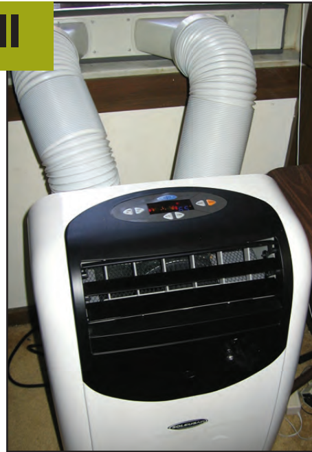
Portable heat pump located in Dulley's home office. Notice the two ducts leading to the window adapter. Source: James Dulley
