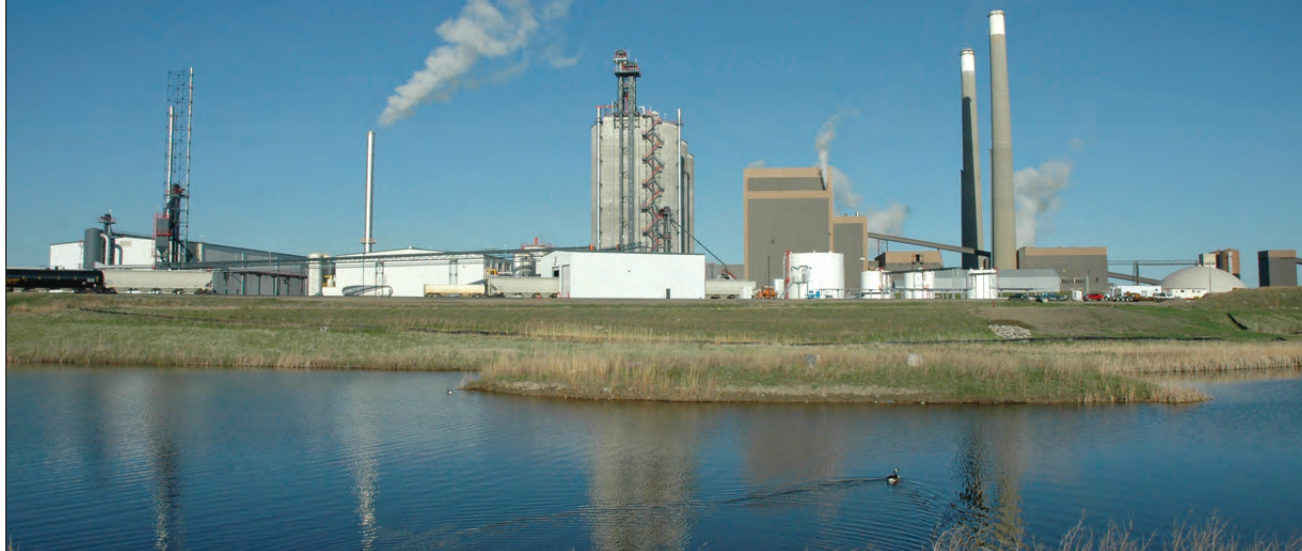
Blue Flint Ethanol uses steam from Coal Creek Station (right) to produce ethanol from corn.
