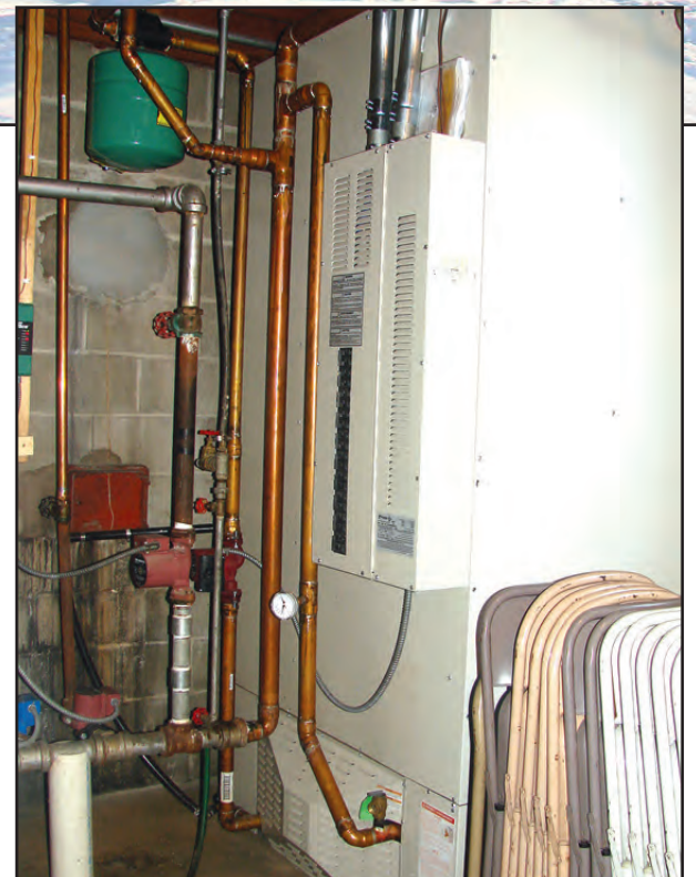
A storage furnace can usually fit well into an existing heating system, whether it's a forced-air or hydronic application.
