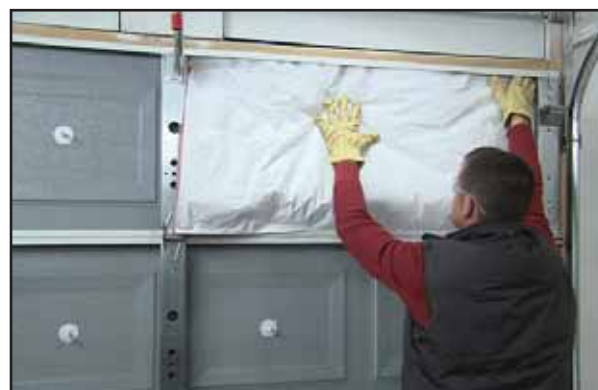
After clips are stuck to garage door, the fiberglass batts are pressed over the clips. Source: Owens Corning
