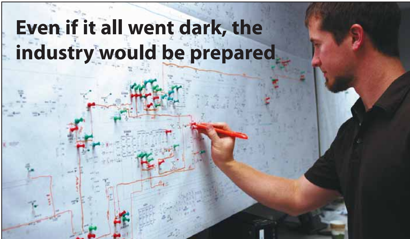
System Operator Cody Smith highlights a transmission line being placed in service. Highlights represent transmission lines and substations that have been returned to service. Green push pins represent open circuit breakers or switches. Red push pins represent closed circuit breakers or switches.
