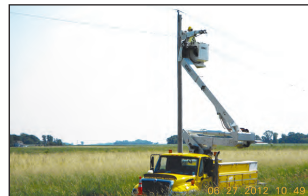
MCPA linemen remove three miles of overhead conductor and poles in Bismarck Township of Sibley County to prepare the way for CapX2020 transmission line project. The overhead line is being replaced with an underground line.
