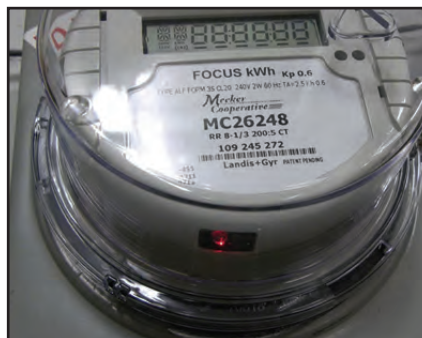
If there is power to the meter, you will see a red light inside the meter, either on the bottom or on the left side, and digital meters will have a numbered display.
