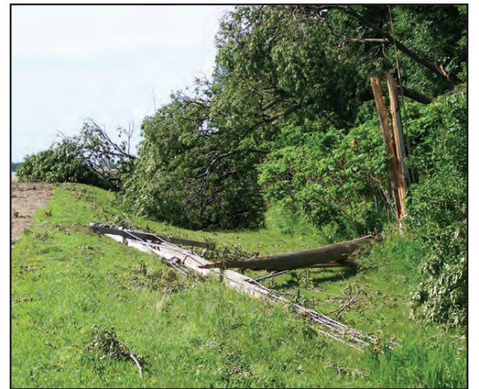
Winds took down this transmission line and pole with the help of trees falling on the line north of Hector.
