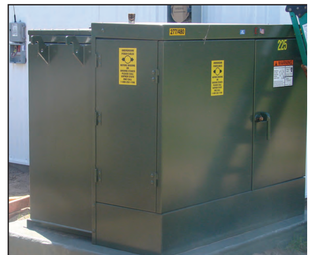
Alpha Foods just added a second generator. During times of control, they keep milking and receive a special electric rate.
