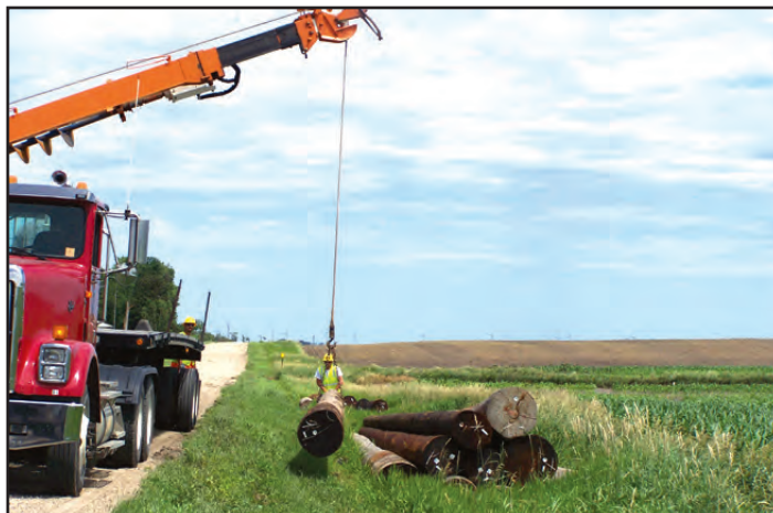
Great River Energy unloads new transmission poles south of the Brookfield Sub. Over 70 new poles will be needed to replace a two-mile stretch of poles destroyed by high winds.
