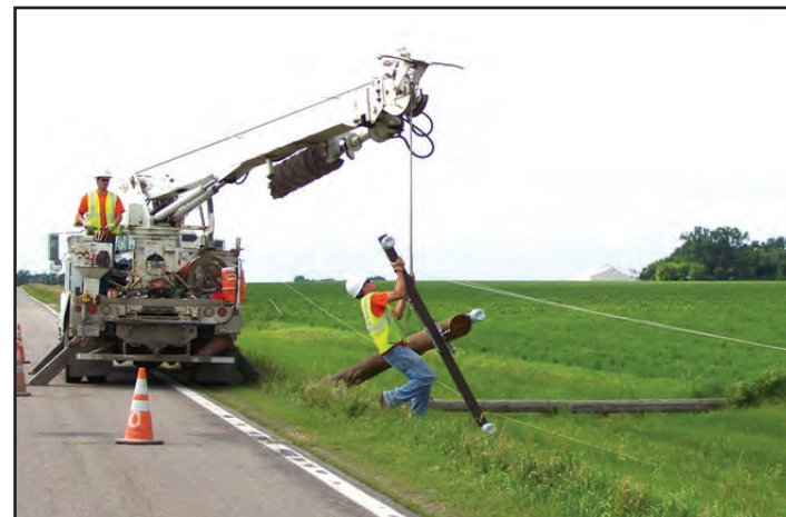
Employees of Legacy Construction of Sauk Center put cross arms and hardware on a new pole south of Hector.
