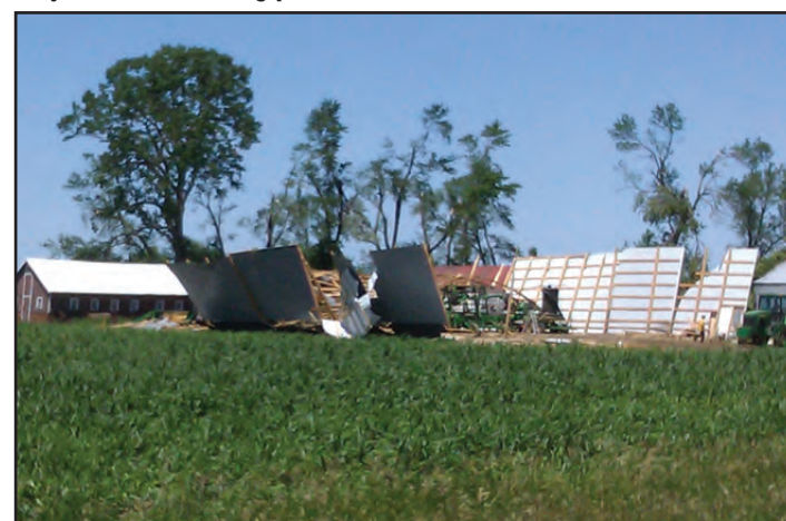
Member's shed damaged by wind.
