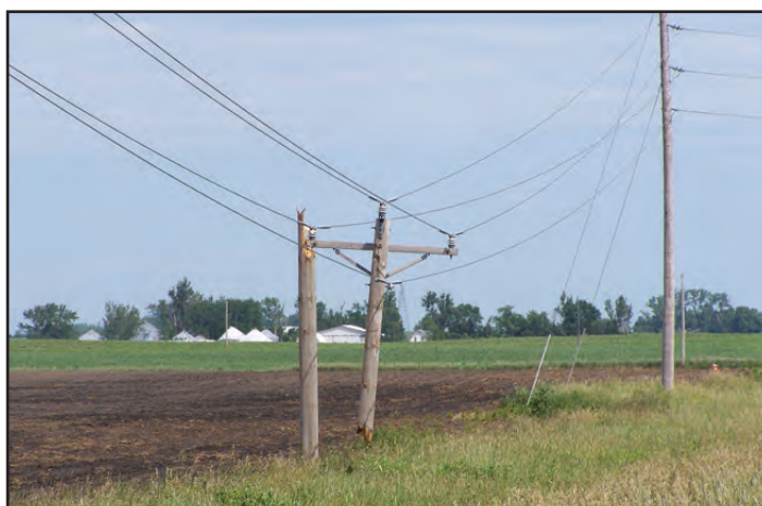
Pole snapped off but was still hanging in line on Hwy. 16.
