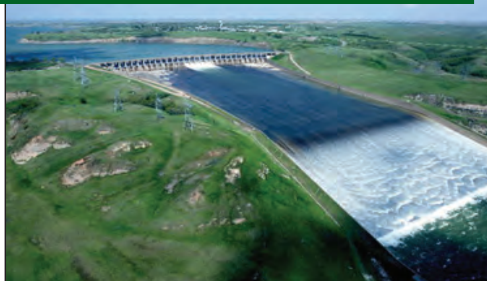
Aerial view of the Garrison Dam upstream of the Bismarck-Mandan, ND area. The dam is releasing water into the Missouri River at a flow of 140,000 cubic feet per second.
