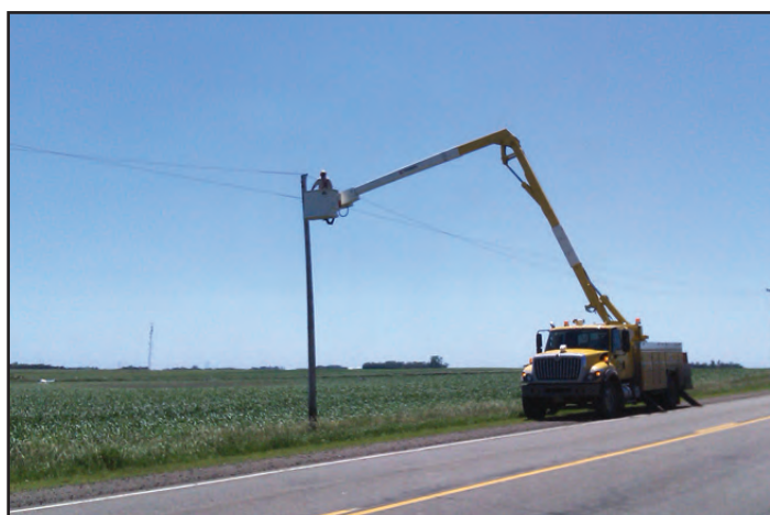
MCPA crews fix wires tangled by the storm.
