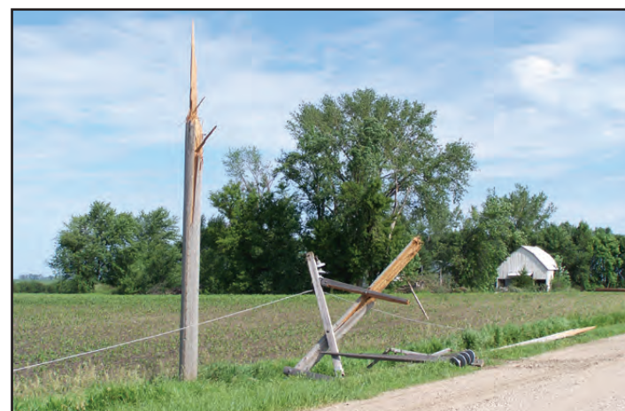
Broken pole north of Hector, one in a line of 70 poles that went down.
