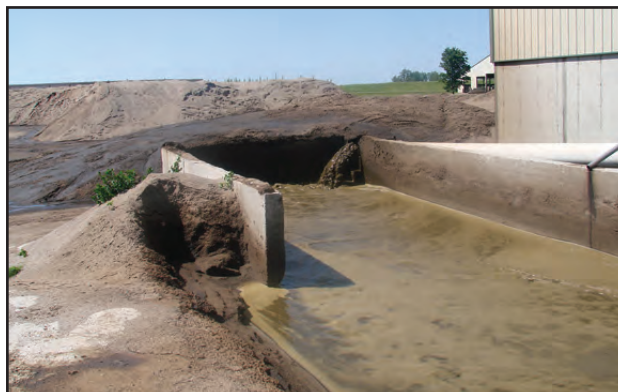
The sand-separation lane run by a variable frequency drive.
