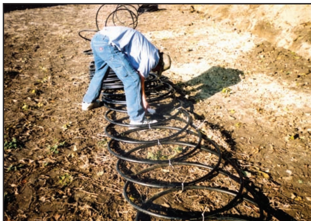
This system uses circular loops to expose heat-collecting liquid to the ground's heat, which is then transferred into the home.
