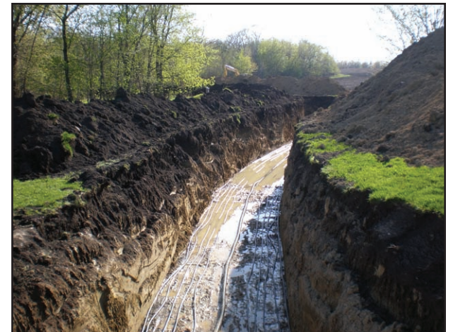
Another system uses a straight loop. Contractors have their preferences. Your cooperative is a good source of information and contractor lists.
