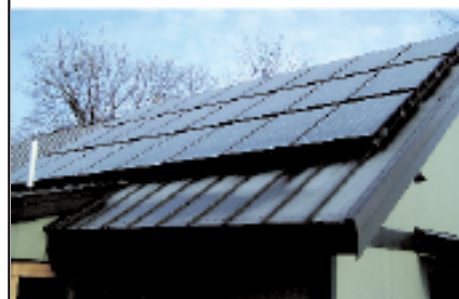
Solar PV System
