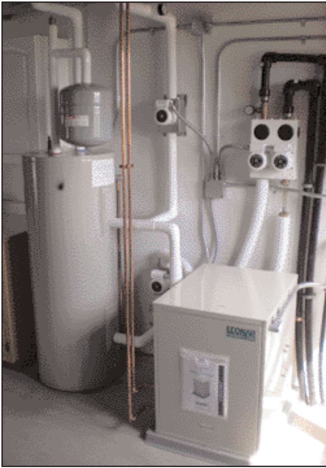
In this home's mechanical room the heat pump unit sits on the floor on the right. It uses hydronic in-floor heat. It is smaller than a standard furnace. If the unit were used on a force air system it would have a furnace fan/air handler and be attached to duct work. In this installation (above), a desuperheater heats domestic hot water using spare heat from the heat pump system.
