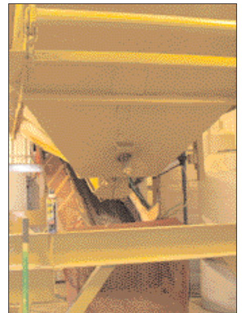
Aggregate stored in bins is discharged onto a conveyer belt and is ready to be mixed according to a predetermined mix design.
