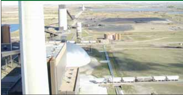
View from roof of Coal Creek Station.
