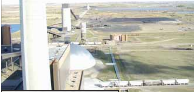
View from roof of Coal Creek Station.
