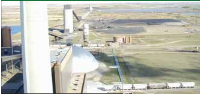
View from roof of Coal Creek Station.
