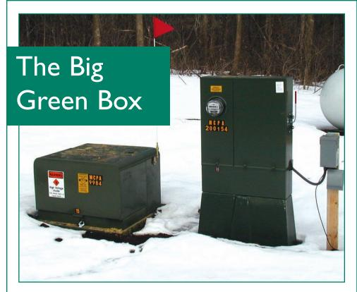
hey're big. They're often green. They generally sit on a concrete or fiberglass base. These electrical boxes are padmount transformers. They do the same job of stepping down voltage like a transformer hanging atop a pole, except they do it for underground services. Developers often put in underground power lines to improve the aesthetics of new neighborhoods. This eliminates utility poles and overhead wires, however it requires the installation of pad-mount transformers in people's yards.
